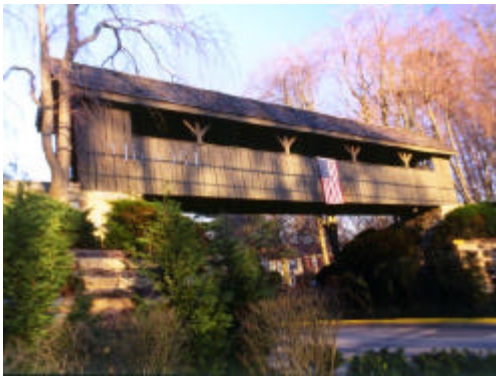
COBBLESTONE, 54', 1984, pedestrian, 46-29-A. Across Hidden Bridge Rd. NW of Pohick, Fairfax County, VA. Pohick Rd. (SR638 changes to SR641) NW about 2 miles from jct with US1 in Pohick to the bridge at the Cobblestone housing development. May, 2003. Photo by Don Burnell.
